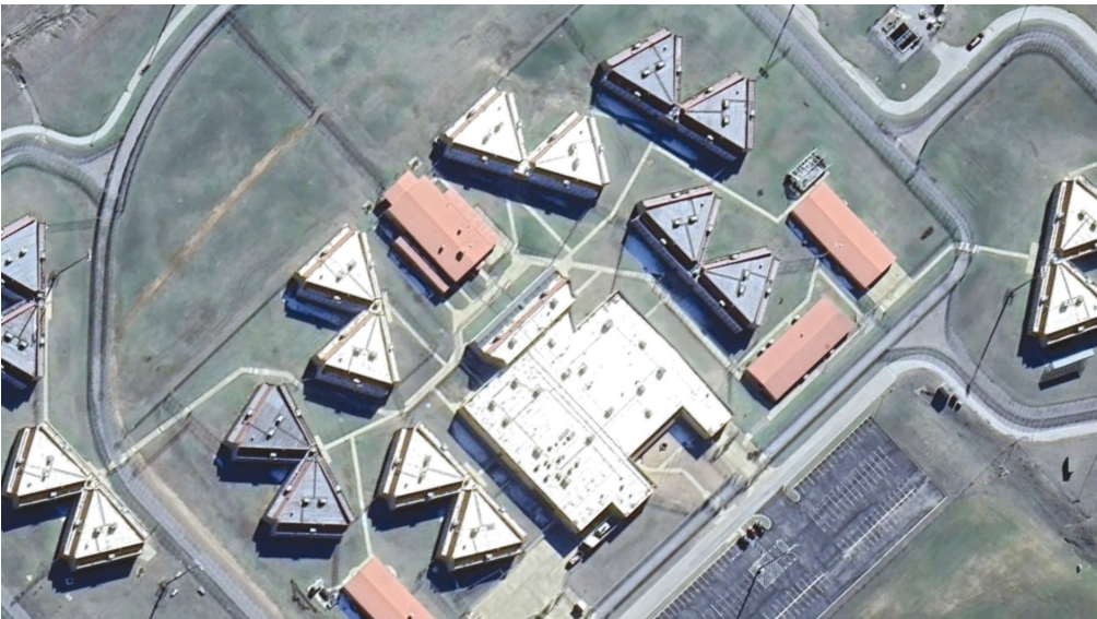
Aerial view of the Watonga ICE facility pre-renovations.
